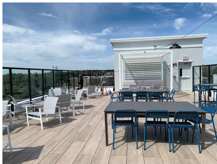
Figure 1: Rooftop deck with high glass guards.
