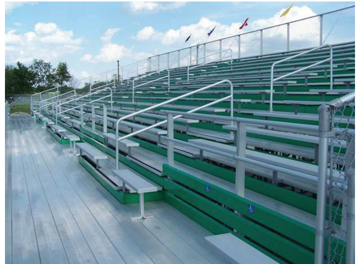
Example of wheelchair space locations in telescopic bleachers.
